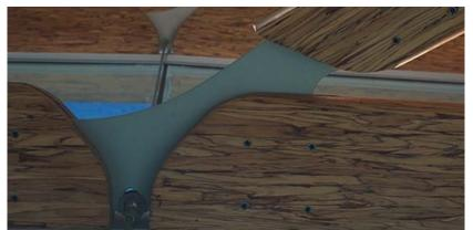
Figure 13: This detail shows the connection of the support arm and muntins to the aluminum plate with (4) tight-fit pins. Also shown is the intersection of the support cable with the aluminum plate.
