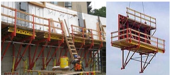
Figure 7: PERI CB 240 climbing platform system (Cradle) Figure 8: Movement to next lift via crane
