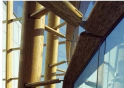
Figure 16: Curtain wall similar to Arena Stage (image provided by StructureCraft Inc.)
