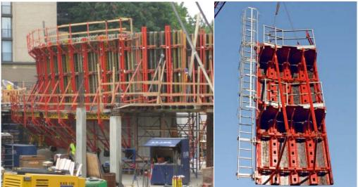
Figure 9: PERI RUNDFLEX formwork prepared for a lift pour Figure 10: Movement to next lift via crane
